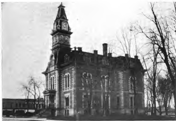
PRESENT CEDAR COUNTY COURTHOUSE
